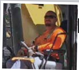
Excavator Operator William Alex Velasco .
