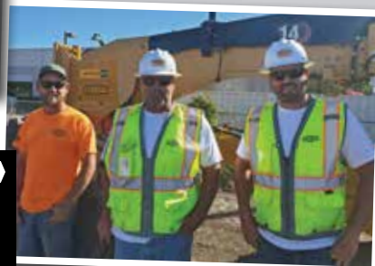
From left: Gradesetter Kevin Todd , Foreman Ken Caselli and Finish Blade Operator Matt Matej work for Ghilotti Construction .
