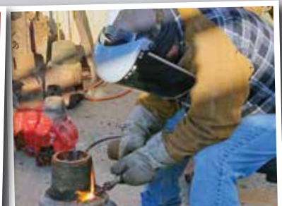
HDR Javier Monroy works for Maggiore Bros. Drilling.
