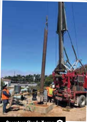
Operators Claude Young and Eduardo Mauricio work for Maggiore Bros. Drilling.
