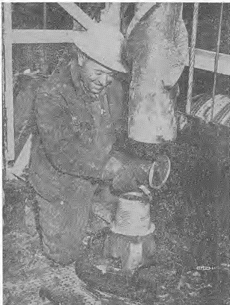
Bro. Arthur F. Collins, Local 3 member, is shown doping threads of the bit before the first section is coupled on. (See picture on page one.) Art is a native of Oregon, now lives at Angels Camp with his family. He began work for Calaveras on Sept. 3, 1945, has operated jackhammer, churn drills, Joy Drill, and now is assigned to the new Bucyrus Erie 50-R.
