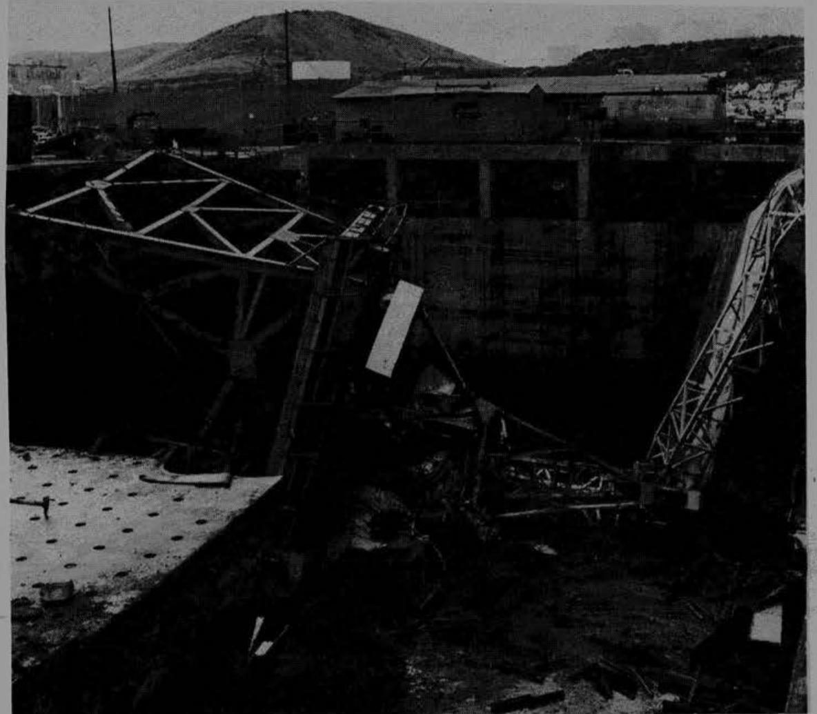
THE ACCIDENT which resulted in the wreckage seen above took the life of a 64-year-old operating engineer from San Pablo, California. This mishap, which happened
